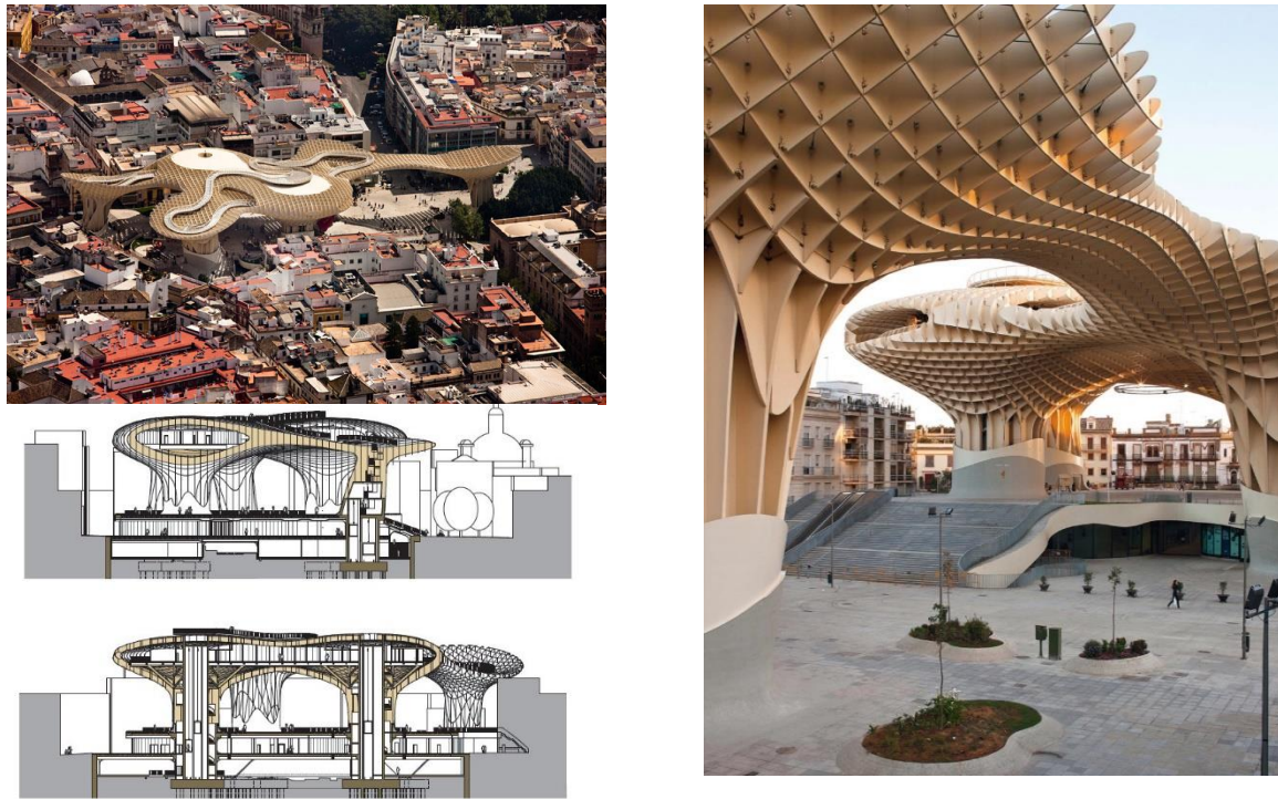
Figure 4. The Metropol Parasol Sevilla building uses parametric design with complex structures (Ashui, 2011)
